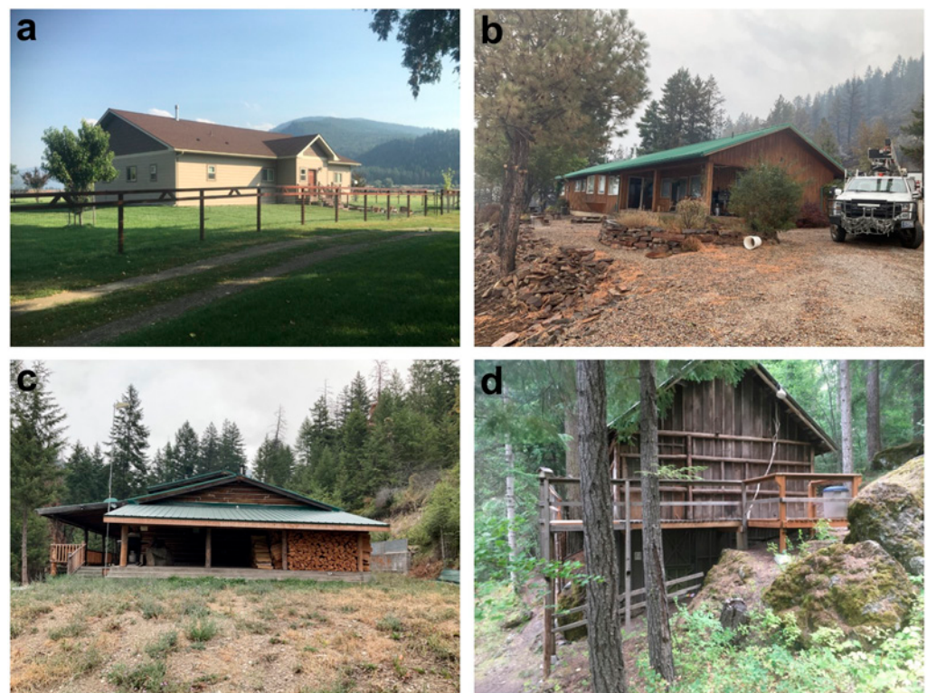
Figure 2. Structure triage categories defined by wildland firefighters during structure triage assessment. Images were obtained from the structure triage dataset [33]. (a) A D-SA structure, with vinyl siding and minimal vegetation in close proximity, which exhibits a very low probability of ignition. (b) A D-PH structure that has adequate defensible space and accessibility but is located on a slope, which may necessitate additional protection tactics. (c) An ND-PL structure which is a log cabin with firewood stacked against the structure, resulting in a substantial risk of ignition. However, it benefits from having minimal vegetation in its immediate vicinity. (d) An ND-RDB structure that presents several concerns, including the presence of overhanging trees, its positioning on a slope, and the use of wood siding, all of which increase the risk of ignition.
