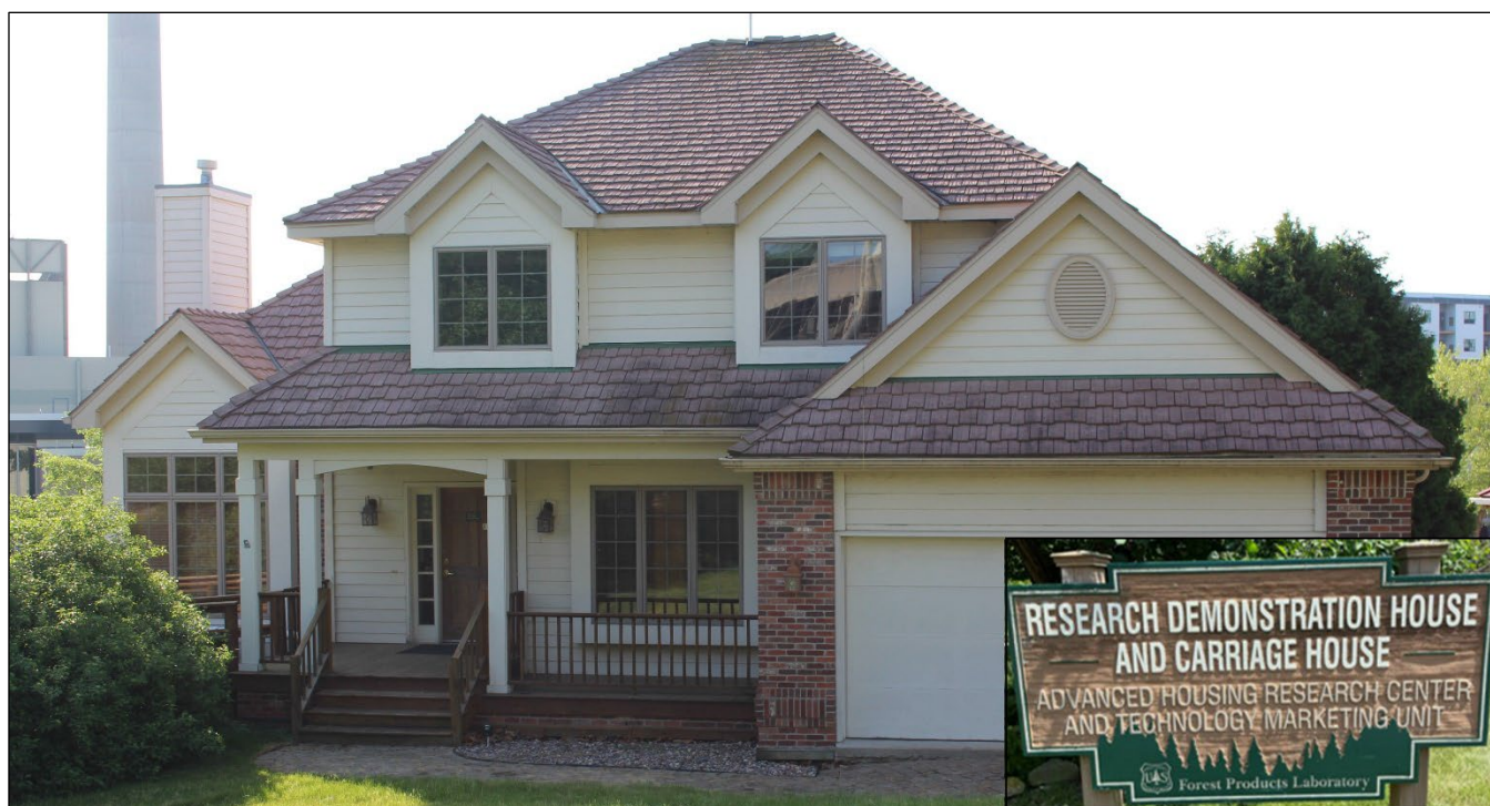
Figure 1—Northern climatic research house (originally called the Research Demonstration House) and the sign that is located near the front of the house (inset photo) (photos property of Mississippi State University, used with permission).
