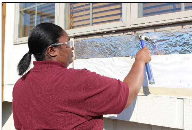
Figure 21—A hammer was used to gently strike the sheathing to probe for decay and deterioration (photo property of Mississippi State University, used with permission).
