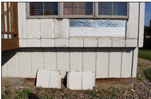
Figure 20—Section of T1-11 siding removed from beneath the triple mullion dining room window (photo property of Mississippi State University, used with permission).
