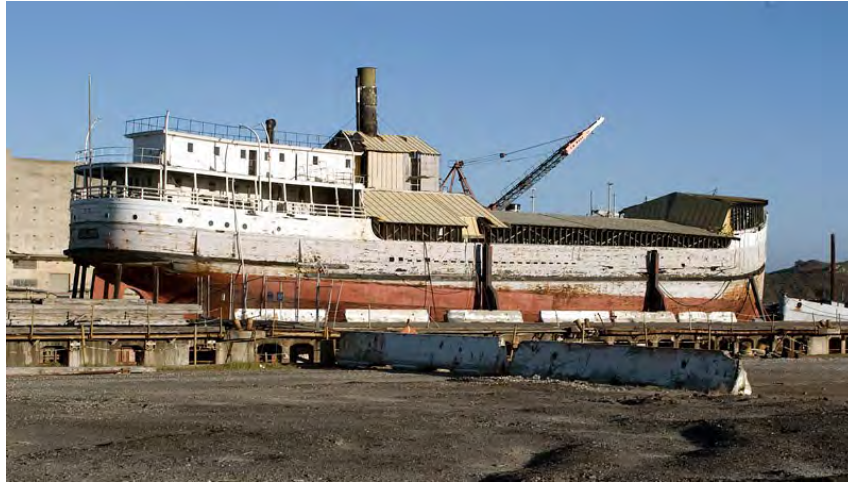
Figure 1 —Wapama placed on a barge at the Richmond Reserve Shipyard in Richmond, California.
