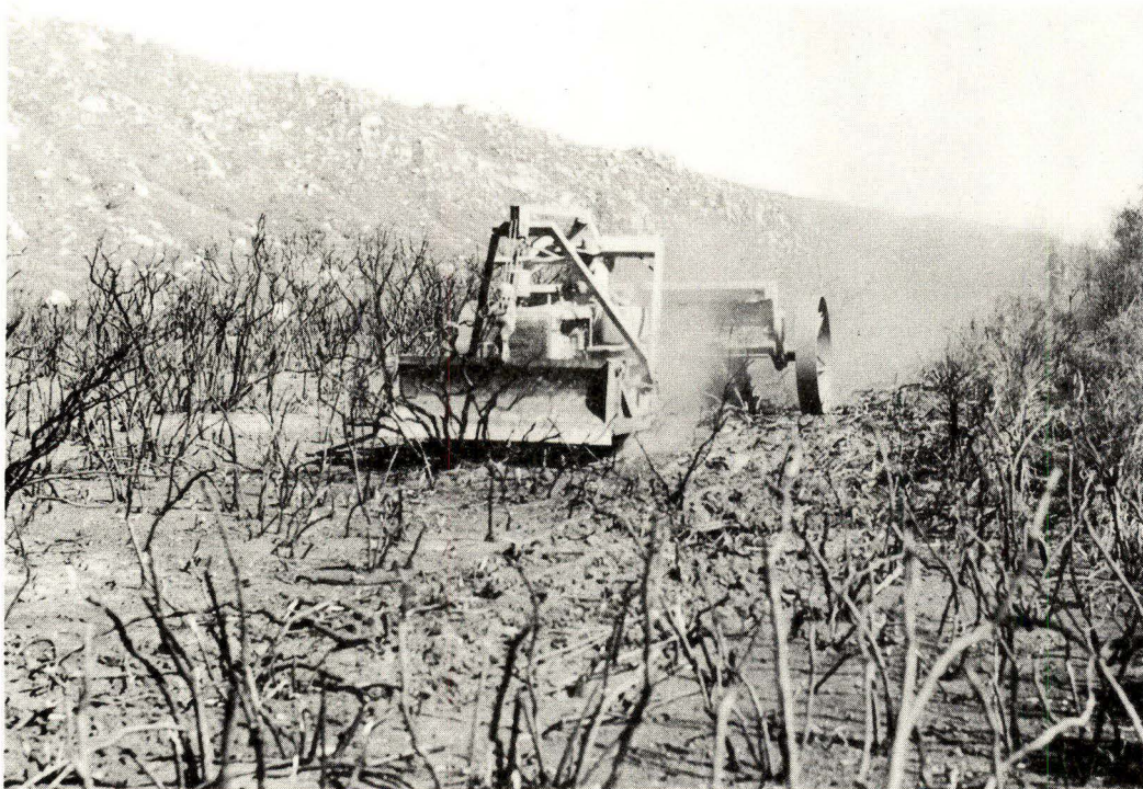
Figure 5.--The rangeland drill is not damaged by small brittle stems such as chamise. The dozer blade is needed, however, to remove tough stems such as the oak in front of the blade.
