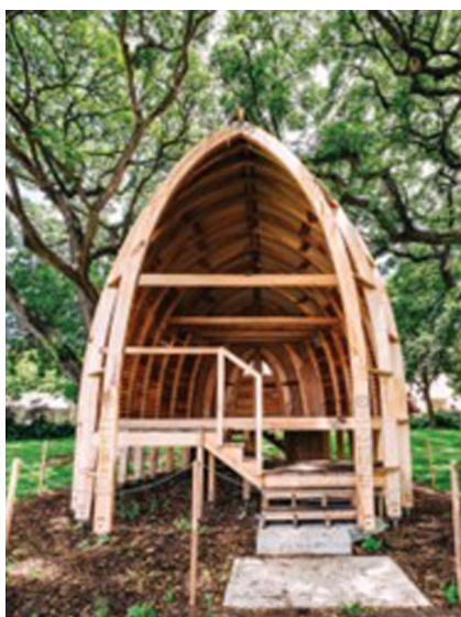
FIGURE 7. Image and front view, of small home, “LIKA,” model constructed with Falcataria falcata lumber on University of Hawai'i at Mānoa campus. Photo credit: The Albizia Project.
