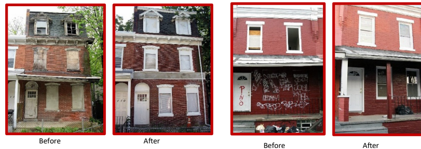
FIG. 3 Vacant and abandoned home remediation examples.
