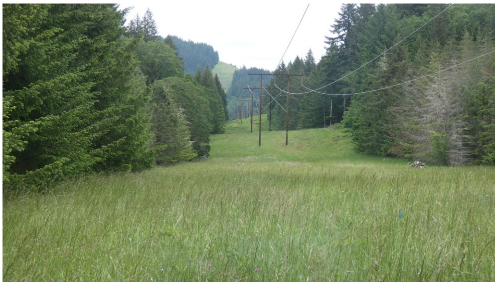
Figure 39—Powerline corridor. USDA Forest Service photo by Bruce G. Marcot.
