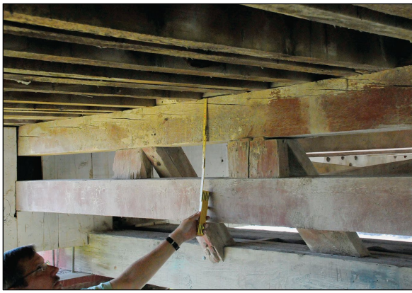
Figure 6.8—Example of using checking in a member to measuring the slope of grain in bridge. The end of the scale points to the start of one check.
