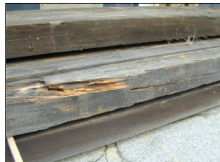
Mechanical damage
