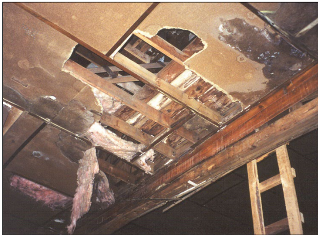
Figure 1.8—Removing the ceiling panels revealed that the fiberglass insulation was saturated with water.
