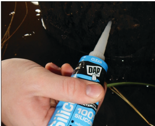
Figure 2.14—Silicone is used to fill the small drilling hole.
