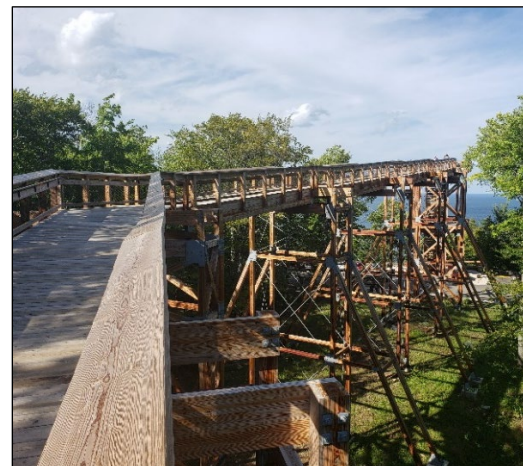
The replacement of Eagle Tower, built with glued-laminated timber, was opened in 2021.
