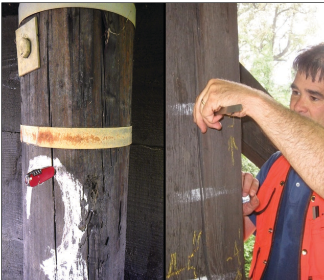
Figure 2.3—Probes are used to assess depth of cracks, checks, and through splits in timber bridge elements.
