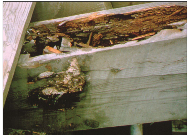
Figure 1.2—Fruiting bodies can indicate extensive damage inside the beam.
