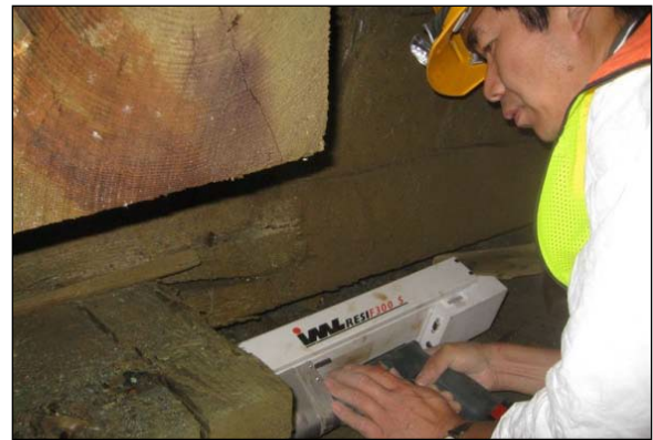
Resistance micro-drilling being performed at a foundation member.
