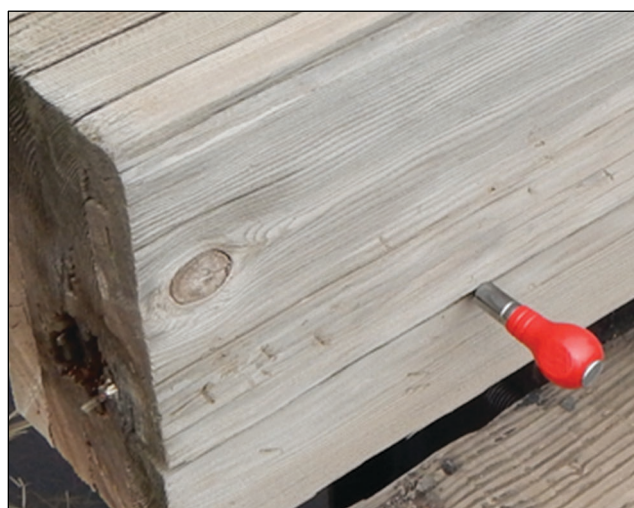
Figure 2.2—An awl is used to assess depth and presence of decay in a horizontal split.
