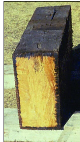
Figure 1.15—Only the outer portion of this timber contains preservatives.
