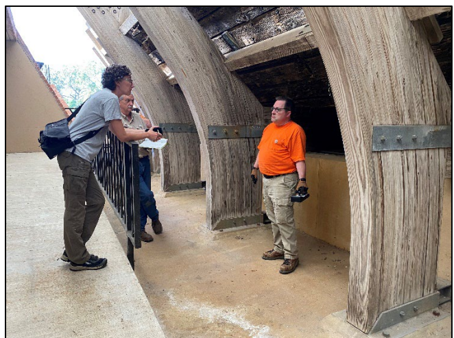
Figure 3—On-site team member discussion of inspection techniques used during the USS Cairo support structure condition assessment.
