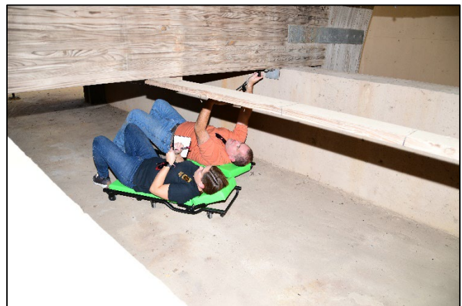
Figure 7—Team members performing moisture measurements of USS Cairo glulam support structure.
