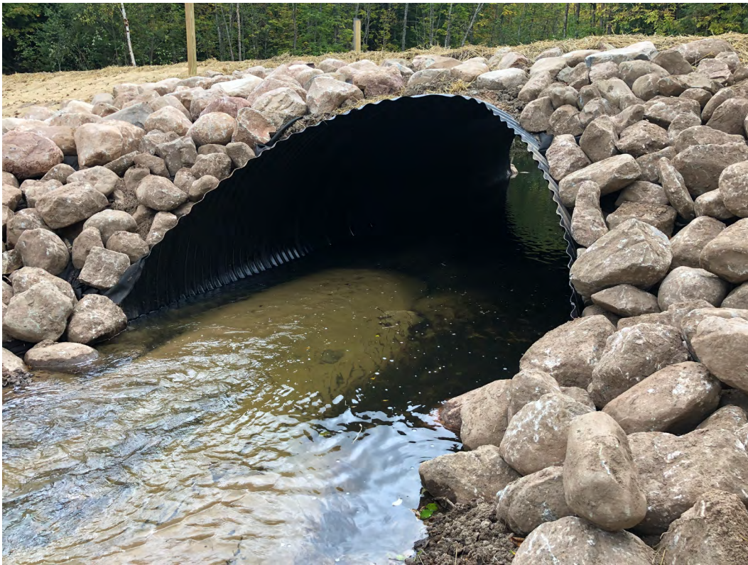
Figure 9. —Newly installed permanent crossing sized to pass floods, debris, and aquatic organisms and designed to last 100 years. USDA Forest Service photo.
