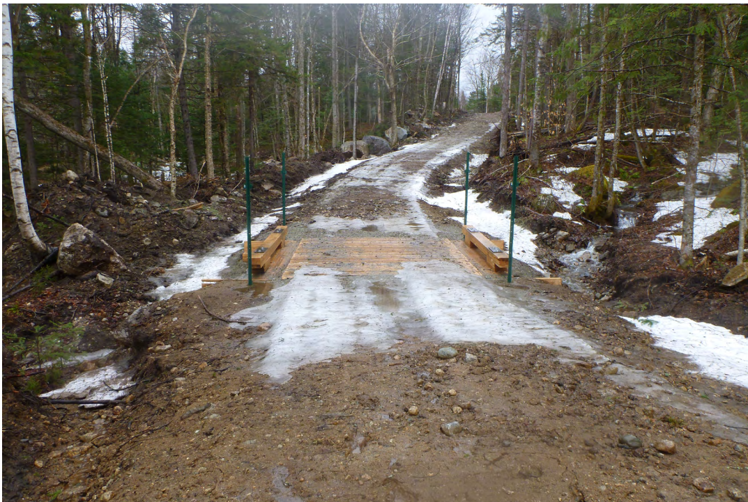
Figure 8. —One example of a temporary bridge crossing for a haul road. USDA Forest Service photo.
