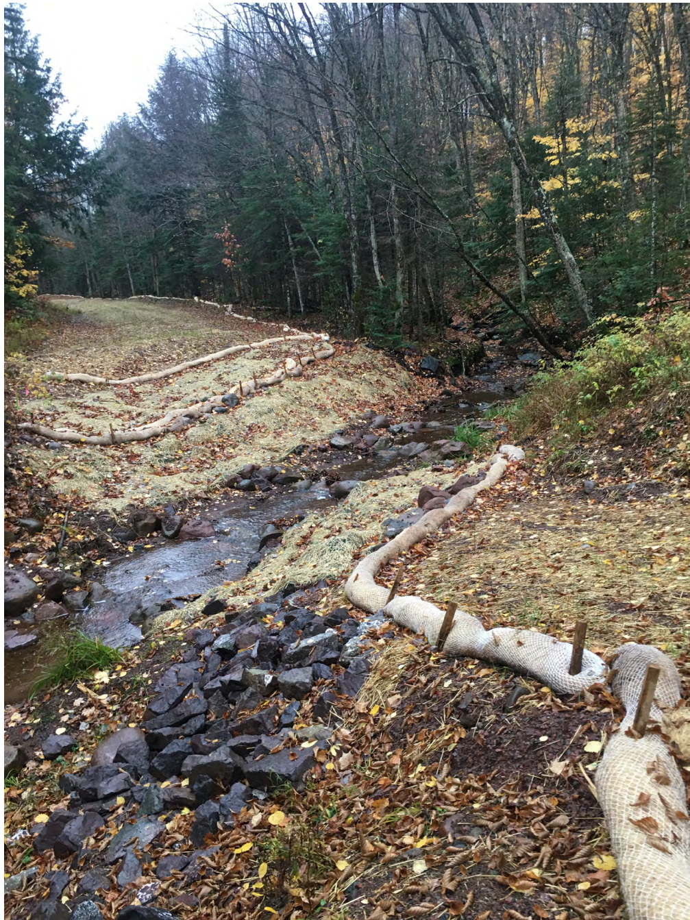
Figure 12. —Crossing removal and stream restoration. USDA Forest Service photo.
