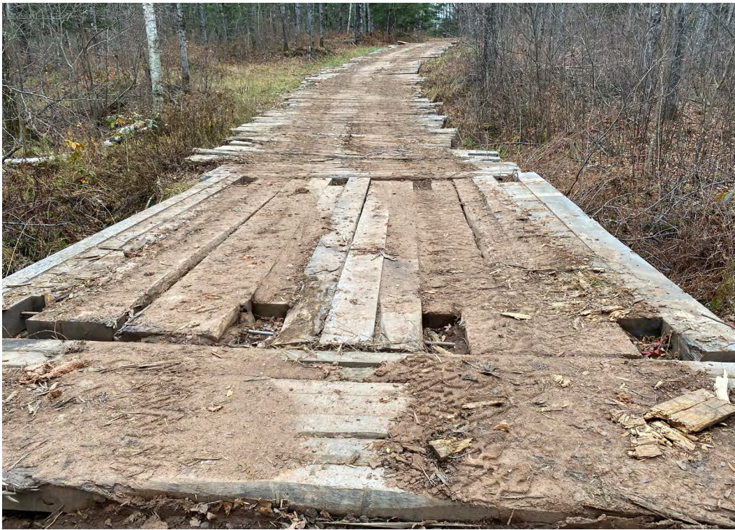
Figure 3. —Timber mats in place protecting soil on a stream crossing and the approach. Courtesy photo by Wisconsin Department of Natural Resources.
