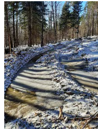
Figure 6. —Water collecting in a forwarder trail during a thaw. This might have been avoided by installing adequate drainage on the downslope side. USDA Forest Service photo.
