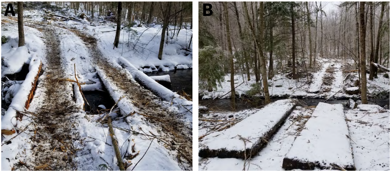
Figure 10. —Temporary timber mat stream crossing (A) installed and in use and (B) removed in preparation for the end of the season. Courtesy photos by University of New Hampshire Extension.
