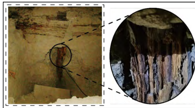
Figure 3 —Photos of 2-2 foundation timber pile under the streamway surface.
