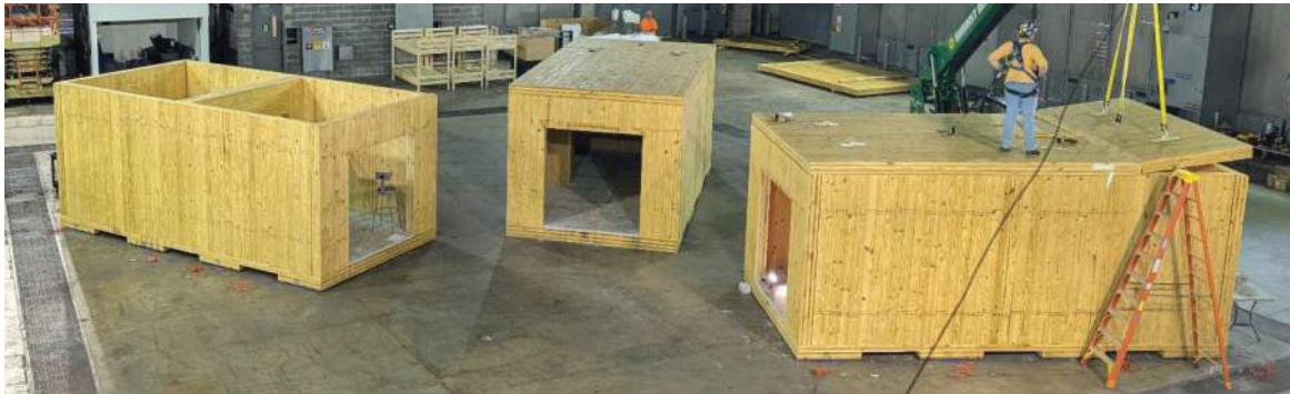
Figure 1: The three test structures during construction all located under the Fire Products Collector. During testing, the structures not being tested were protected with gypsum board and ceramic batting on the exposed exterior.
