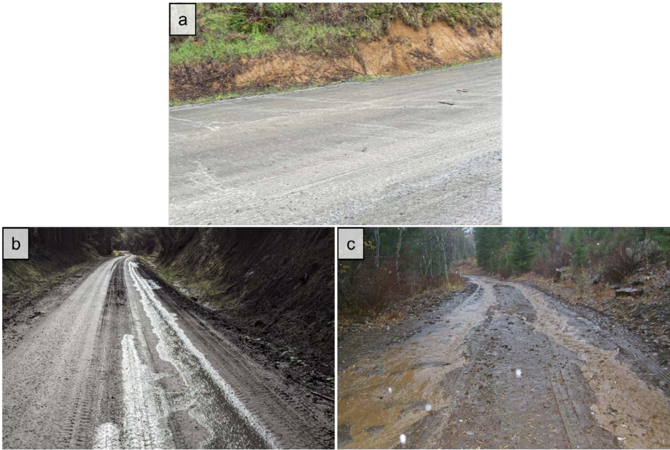
FIGURE 2 | Example photos of (a) an un-rutted road with flow heading to the ditch line from the centre of the road; (b) water travelling down-road in a wheel rut instead of being directed to the roadside ditch; and (c) a heavily rutted road with channelised, sediment-laden flow heading down-road. The road widths seen in each of these photos are approximately 5 m.
