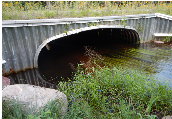
A stream simulation crossing at the Chequamegon-Nicolet National Forest that did not overtop during the 2016 flood. USDA Forest Service photo by Dale Higgins.
