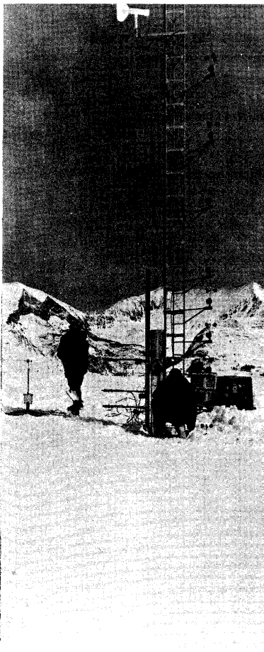
R. A. Schmidt, Jr., and R. D. Tabler, developing models of sublimation for blowing snow control. Schmidt (right), calibrating a snow particle counter; Tabler (above), observing snow depth behind an experimental snow fence, near Laramie, Wyoming.
