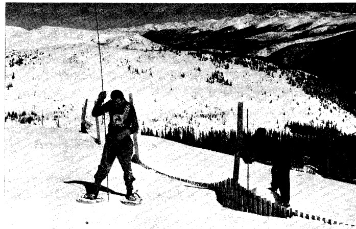
(Upper right) Building snowfence near Loveland Pass, Colorado, to help keep blowing snow out of an avalanche path; (below) R. W. Hanson and R. E. Stillman, determining snow accumulation on each side of a snow fence.
