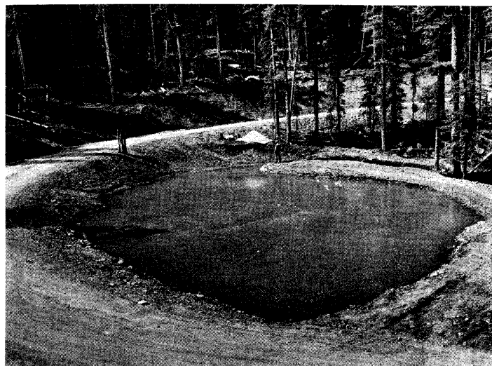
A sediment basin of \frac{1}{4} acre-foot capacity was constructed in 1951 immediately below the stream-gaging station. Annual sediment yield from the watershed following logging averaged only 1.5 cubic feet per acre, net volume.
