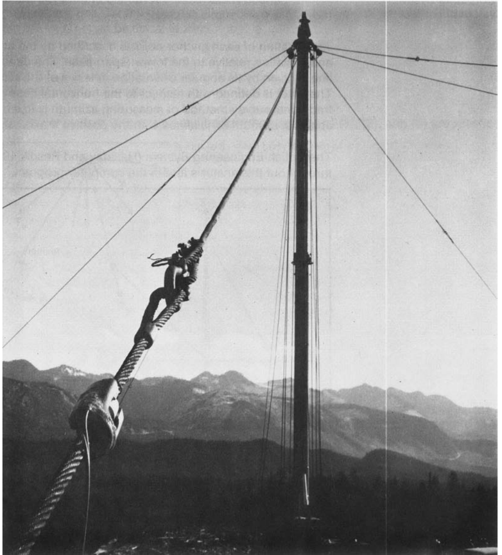
Figure 1—Guylines supporting a steel logging tower.
