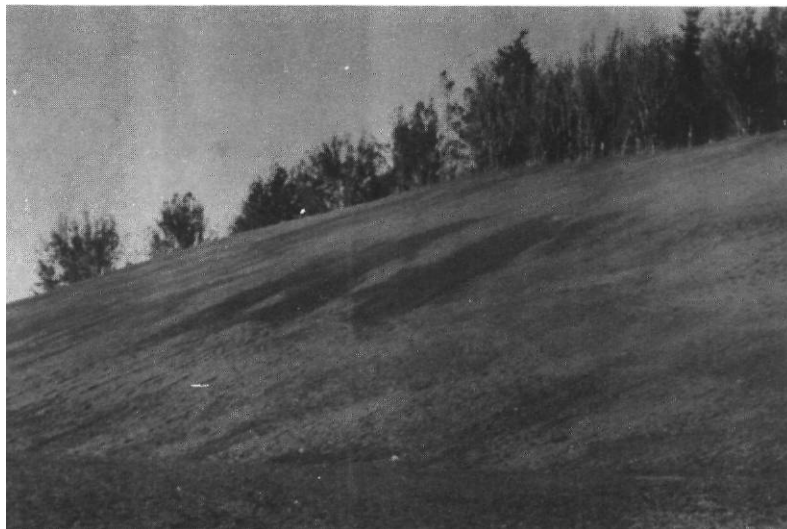
Figure 7.--Piping. Water piping from a road cut or structure shows that free flowing water is being concentrated along open pore spaces within the soil mantle or road prism material. This may indicate the presence of a water table at least as high as the point of exit. It may also indicate a confined zone of concentrated flow under substantial hydrostatic head.
