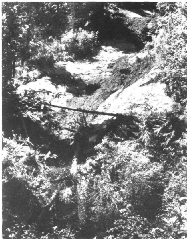
Figure 23.--Failure from accelerated weathering of soil material. Natural weathering of the bedrock does not occur at a uniform rate across a slope. Some spots are weaker (fault zones for example) and form a depression where ground water accumulates. These processes hasten weathering and usually form incipient drainages. Over geologic time, weathered material (soil) or colluvium will slide or wash out. The light areas along the channel in this photo are exposed bedrock surfaces from which soil has been removed by slumping. Note accumulations of soil and debris in the channel bottom. This figure shows how areas shown in figures 9 and 17 look after failure. A "slickrock chute" remains after soil material is removed.
