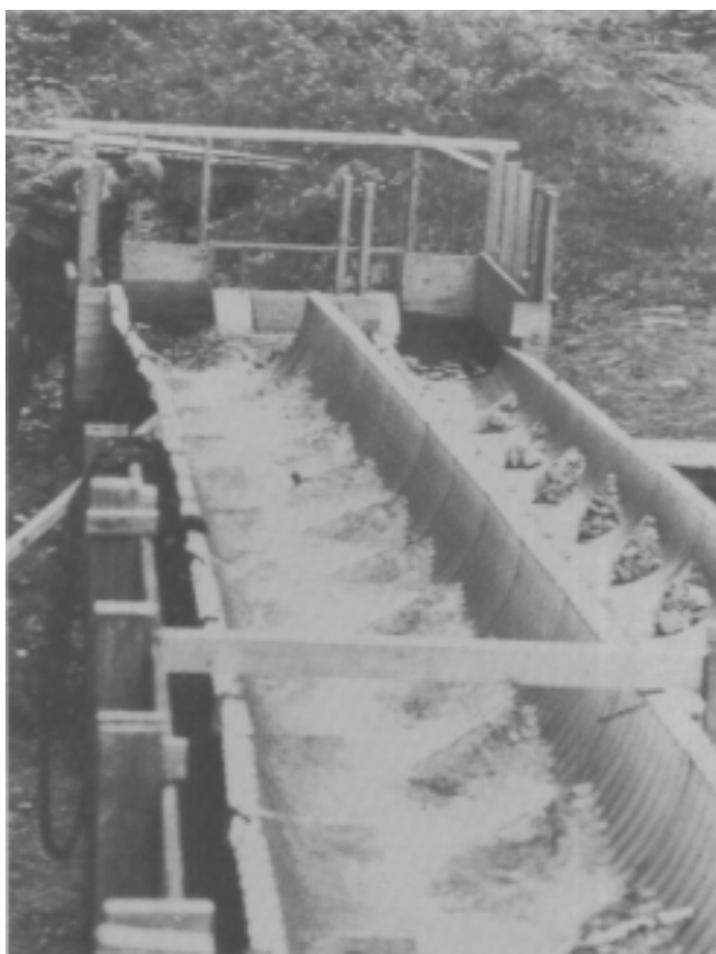
Figure 1.—Baffle culvert installation.
