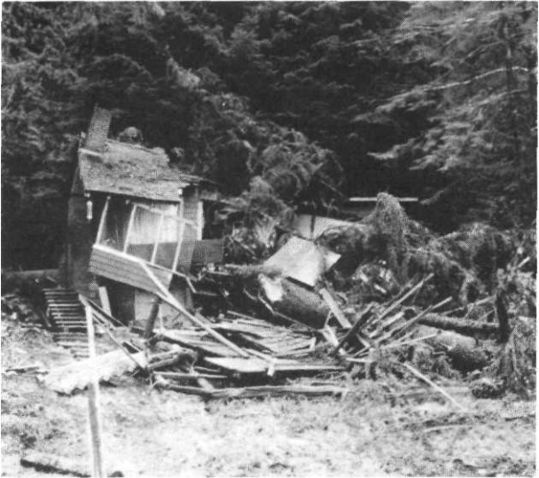
Figure 7.—Damage to recreation facilities caused by a windthrown tree. Decay associated with an injury had weakened the tree.
