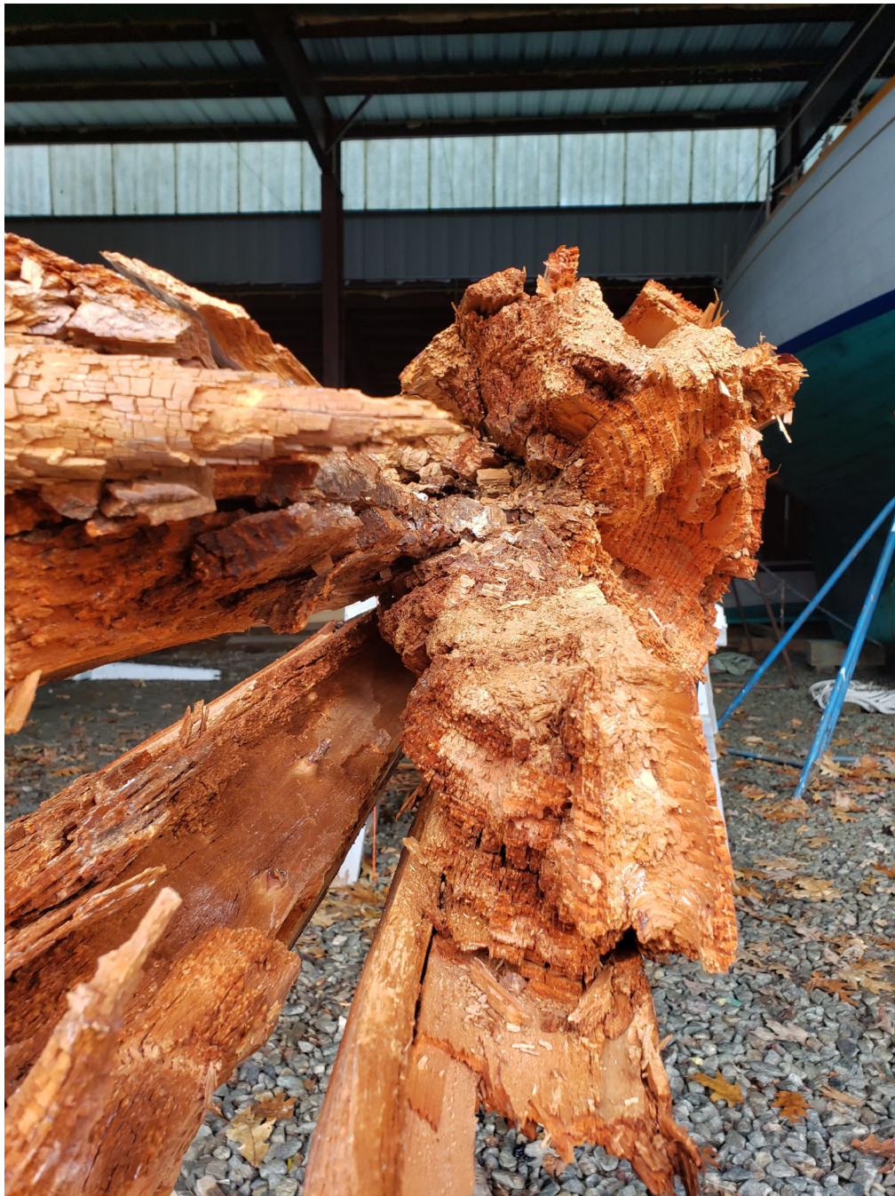
Figure 1E. —Close up of fractured cross section of the Grace Bailey mast. Forest Service photo by Xiping Wang.
