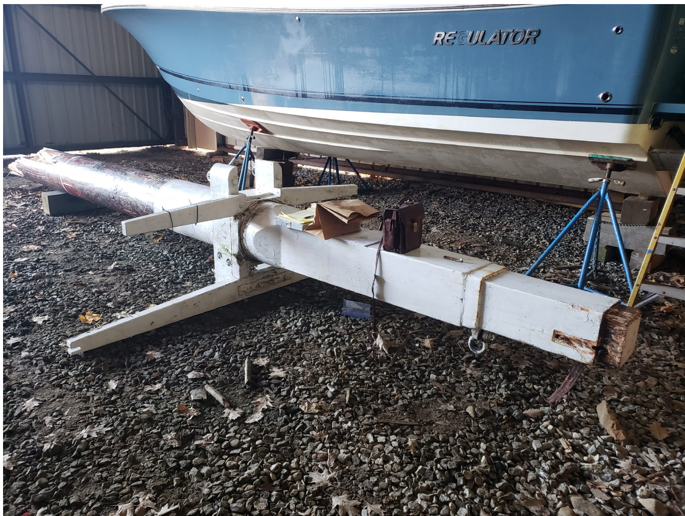
Figure 1A. —Broken top of the Grace Bailey mast. Forest Service photo by Xiping Wang.
