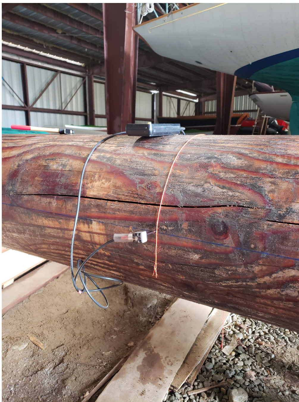
Figure 1J. —Stress wave transmission test performed on the Grace Bailey mast at 21 ft detecting possible internal decay. Forest Service photo by Xiping Wang.
