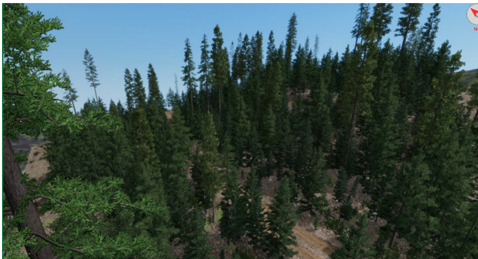
Figure 4.30 —An aerial image of a stand conforming to existing condition Type 5.
