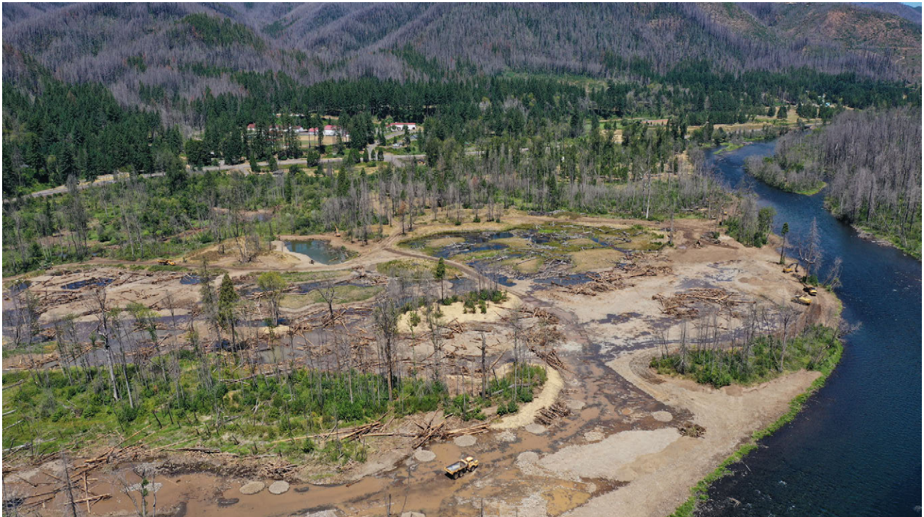
Figure 15—Hauling wood and moving sediment along the McKenzie River floodplain valley-bottom reset project at Finn Rock reach, Willamette National Forest, OR in 2022. Courtesy photo by McKenzie River Trust/Steve Smith Photography.
