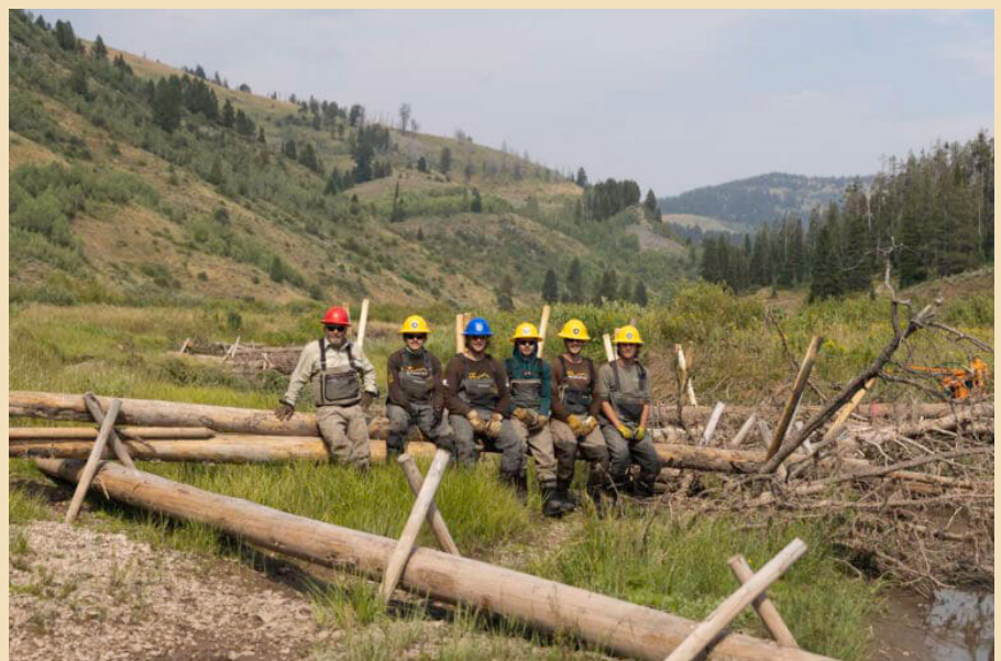
Figure 7—Forest Service and Wyoming Conservation Corps work on Tincup Creek on the Caribou-Targhee National Forest, ID, where the placement of large spreads water and sediment across the floodplain and improves fish habitat, reconnects the channel and floodplain to groundwater, and improves local wildfire resistance. Undersized culverts were also replaced to restore natural flows of water and sediment within the valley. Courtesy photo by Trout Unlimited.
