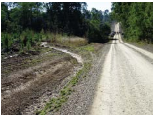
Figure 4.29—Leadoff ditches to allow for runoff discharge into the forest before it reaches a live stream or to avoid water concentration along the road. Photos by Gordon Keller.
