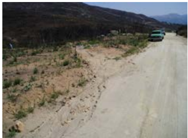
Figure 4.29—Leadoff ditches to allow for runoff discharge into the forest before it reaches a live stream or to avoid water concentration along the road. Photos by Gordon Keller.
