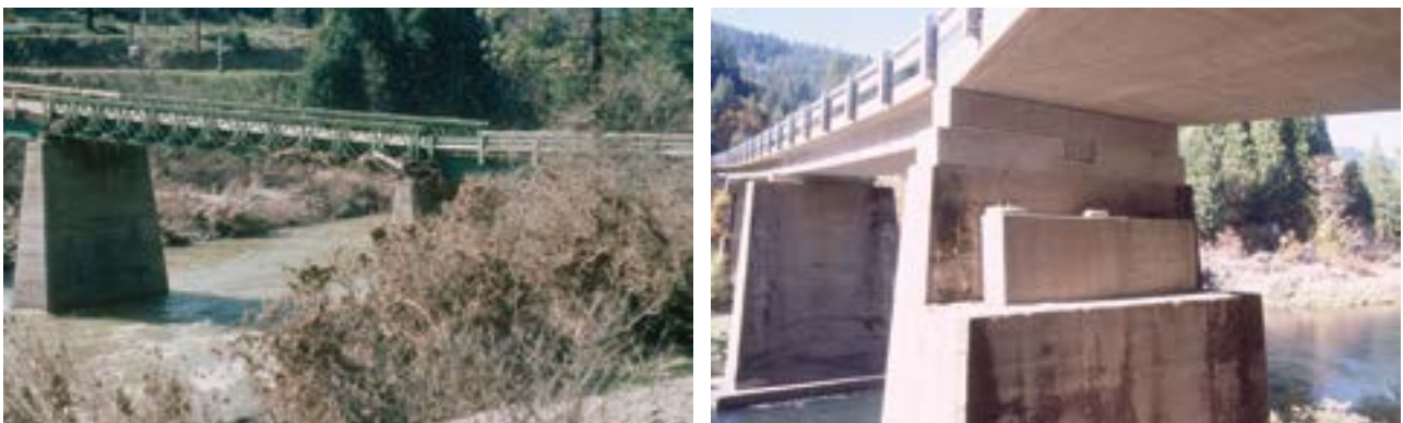
Figure 4.51—Bridge with flood debris in the superstructure and marginal freeboard (left). Bridge abutments, piers, and deck were raised (right) to add freeboard and flow capacity. Photos by Gordon Keller.
