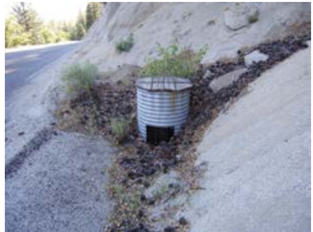
Figure 4.32—A variety of culvert cross-drain drop-inlet structures used on forest roads. Left photo, USDA Forest Service, National Technology and Development Program; right photo courtesy of Gordon Keller.
