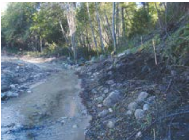
Figure 4.18—Ruts and erosion in the road surface due to lack of surface drainage and maintenance. These roads are particularly susceptible to damage from any storm when in this condition. Left photo courtesy of Joshua Direen; right photo courtesy of Vincent Barandino, USDA Forest Service, National Technology and Development Program.
