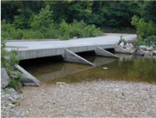
Figure 4.48—Large, vented fords that are resilient and have a predominantly natural stream channel bottom, ideal for aquatic organism passage. High flows can pass readily over the structure, while the natural channel bottom enables aquatic organism and fish movement. Left photo courtesy of Kim Clarkin, right photo courtesy of Terry Warhol.
