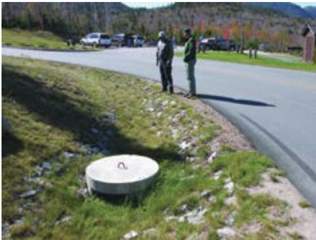
Figure 4.32—A variety of culvert cross-drain drop-inlet structures used on forest roads. Left photo, USDA Forest Service, National Technology and Development Program; right photo courtesy of Gordon Keller.
