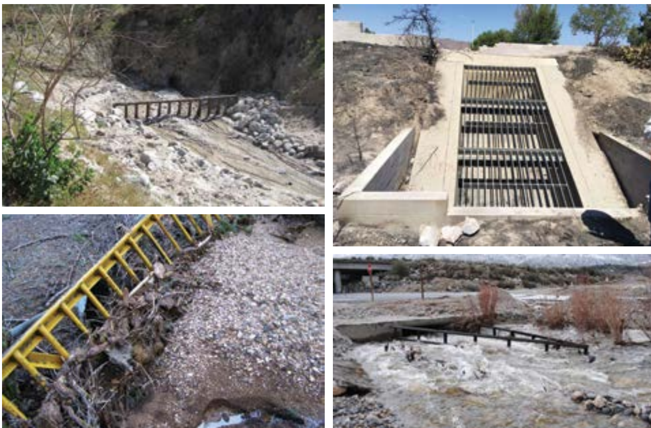
Figure 4.40—A variety of trash racks used in California forests to prevent culvert plugging from upstream sediment and debris. Upper left photo by Allen King, upper right photo by Donald Lindsay, lower left photo by Gordon Keller, lower right photo by Vincent Barandino, USDA Forest Service, National Technology and Development Program.
