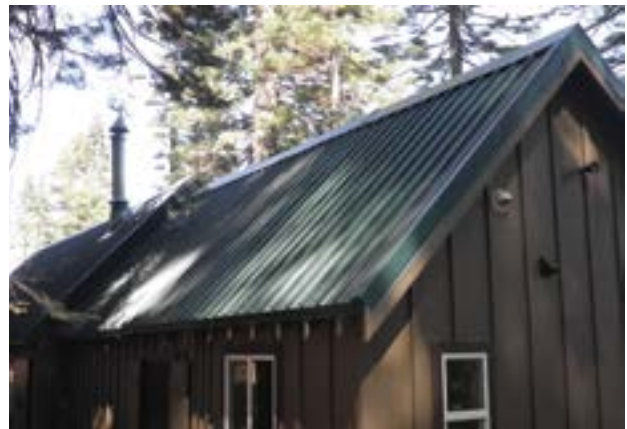
Figure 4.76—Tree thinning for defensible space, metal roofing, and nonflammable siding materials help make facilities more resilient to wildfires. Note that for fire safety, a couple of the trees nearest the structures can be removed. Photos by Gordon Keller.
