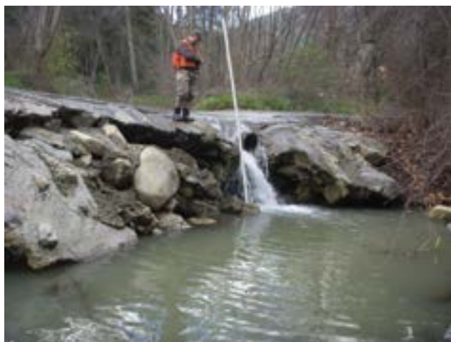
Figure 4.47—A ford damaged over time on Trabuco Creek, Cleveland National Forest, from downstream scour, or structure undermining. Upstream and downstream cutoff walls are typically needed to protect the structure. Photos courtesy of Kirsten Winter.
