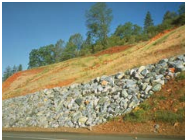
Figure 4.64—Slope stabilization structure types: a rock buttress (left) and an old masonry rock retaining wall (right). Left photo by Gordon Keller; right photo by Joshua Direen, USDA Forest Service, San Bernardino National Forest.
