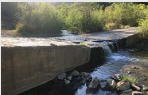
Old ford and dam structures that have been damaged periodically and created barriers to fish and other aquatic organisms. Photos show the Trabuco Creek old ford (left) and Silverado Creek Dam #7 (right) before removal.
