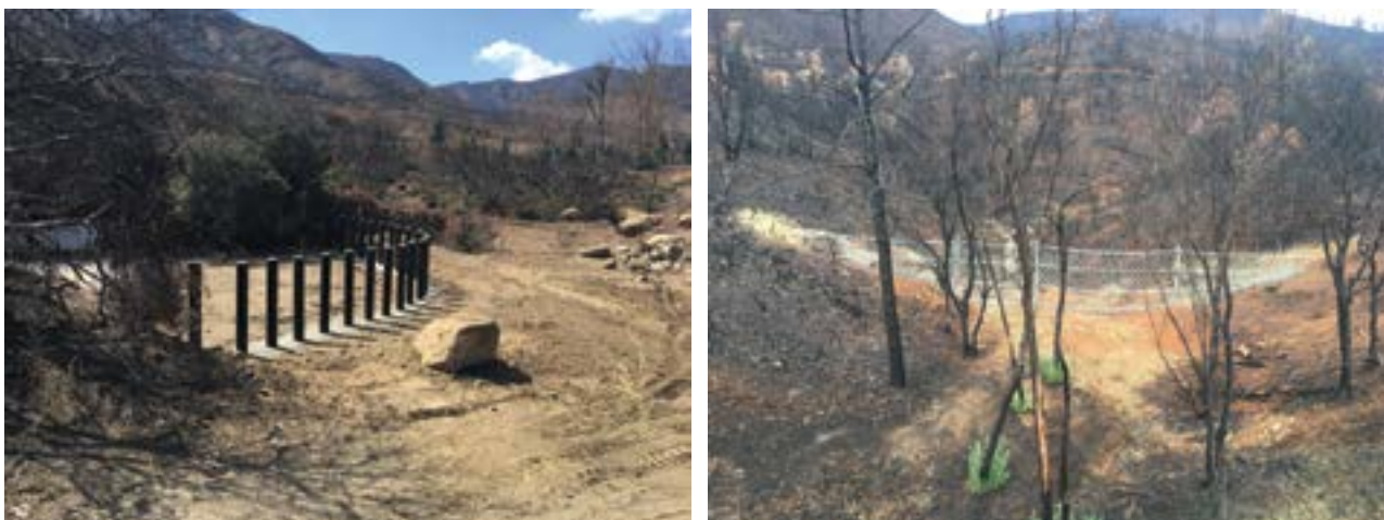
Figure 4.15—Examples of debris-flow adaptation measures, including the installation of bollards (left) in a channel to trap large debris and a debris retention structure using a ring-net (right). Photos by Donald Lindsay.
