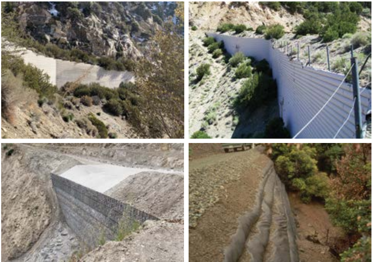
Figure 4.65—Mechanically stabilized earth (MSE) walls: (top) reinforced earth system wall built on the Angeles Crest Highway, Angeles National Forest, in 1972; (bottom left) welded wire MSE wall; and (bottom right) geotextile wall. All were used because they are relatively low cost and easy to construct. Upper photos courtesy of The Reinforced Earth Company; lower left photo by Joshua Direen, USDA Forest Service, San Bernardino National Forest; lower right photo by Gordon Keller.
