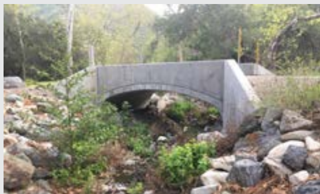
Newly constructed bridges and bottomless-arch culverts that have enhanced fisheries habitat and demonstrated to be resilient to flooding and debris flows. Photos show the Trabuco Creek crossing #3 after bridge construction (left) and Holy Jim #1 with a new bottomless arch (right).
