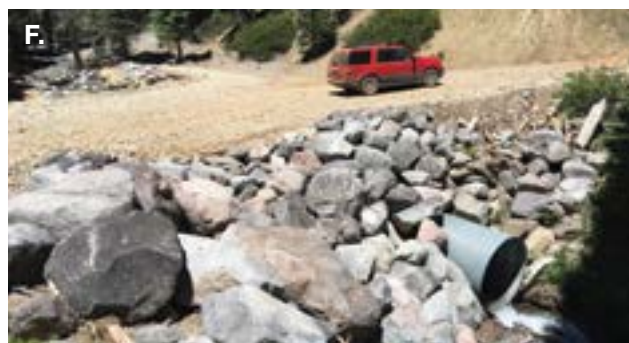
Figure 4.39—(A) Undersized culvert fitted with armored overflow dip to pass water without stream diversion or fill washout. (B) Stream diversion due to a plugged culvert crossing, sending water down the road instead of its natural channel and (C) causing considerable offsite damage. (D) Gabion mattress, (E) turf-reinforcing mats, and (F) rock riprap used to protect an embankment from overflow damage. Drawing adapted from Furniss et al. (1997). Upper photos by Mark Russell, USDA Forest Service, National Technology and Development Program; lower photo by Donald Lindsay.
