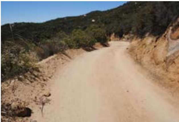
Entrenched bathtub section (common but poor practice)
