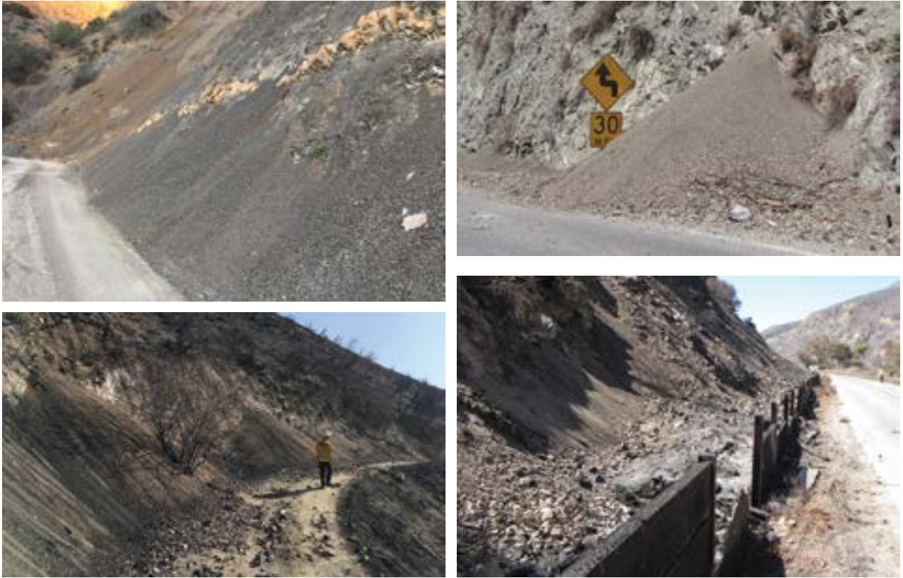
Figure 4.69—Examples of slope ravel from steep slopes and erosive soils or fractured rock, particularly after a fire where vegetation is burned off. Bottom right photo shows a wood retaining structure (which is burned) used to catch slope ravel and rockfall. Top photos by Gordon Keller, lower left photo by Donald Lindsay, lower right photo by Allen King.
