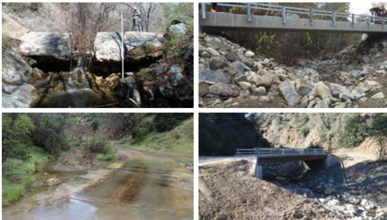
Figure 4.44—Examples of stream restoration projects for aquatic organism passage on Trabuco Creek, Cleveland National Forest (top), and Davy Brown Creek, Los Padres National Forest (bottom). Left photos show the previous barriers to fish passage, and right photos show the bridges constructed to promote fish passage. The bridges are also more resilient to major stormflows. Upper photos courtesy of Kirsten Winter, lower photos courtesy of Kristie Klose.
