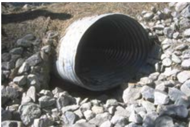
Figure 4.37—Problematic culverts as a result of piping under the structure (left) or loss of capacity from infilling with sediment. These culverts have a high risk of failure, particularly during major storms. Left photo by Gordon Keller, right photo by Donald Lindsay.
