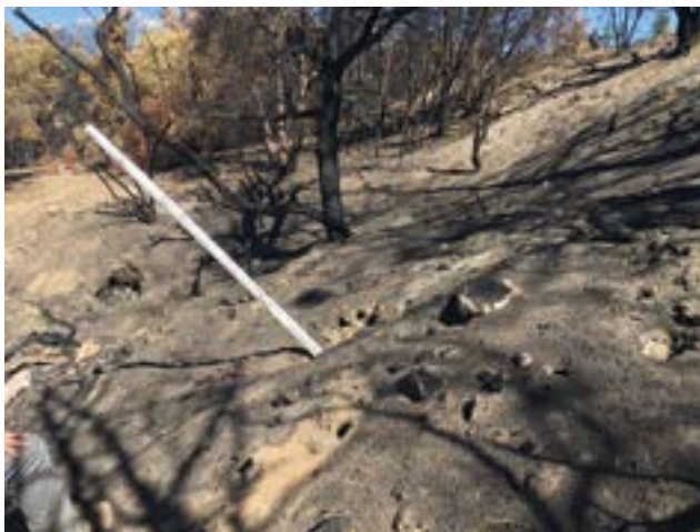
Figure 4.79—An earthen embankment of a dam where wildfire has burned the vegetation and tree roots, leaving deep voids in the embankment. This increases the risk of piping and dam failure, which can be mitigated by removing large vegetation from the dam face and embankments. Photos courtesy of Jonathan Berry.
