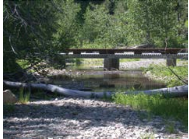
Figure 4.48—Large, vented fords that are resilient and have a predominantly natural stream channel bottom, ideal for aquatic organism passage. High flows can pass readily over the structure, while the natural channel bottom enables aquatic organism and fish movement. Left photo courtesy of Kim Clarkin, right photo courtesy of Terry Warhol.
