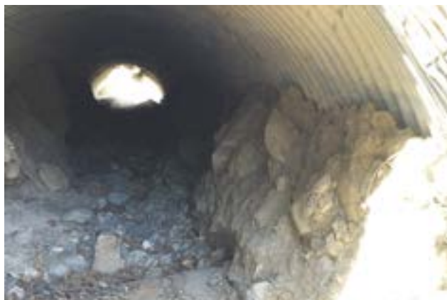
Figure 4.37—Problematic culverts as a result of piping under the structure (left) or loss of capacity from infilling with sediment. These culverts have a high risk of failure, particularly during major storms. Left photo by Gordon Keller, right photo by Donald Lindsay.
