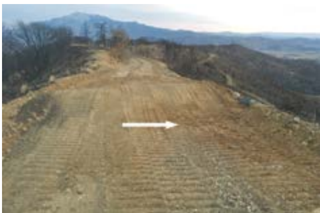
Figure 4.25—Installation of typical rolling dip cross drains on roads. Rolling dips are commonly used on forest roads to remove water off the road surface. They can also be used as a dip to prevent stream diversion down the road and direct flow back into the natural drainage. Left photo by Joshua Direen, USDA Forest Service, San Bernardino National Forest; right photo by Gordon Keller.
