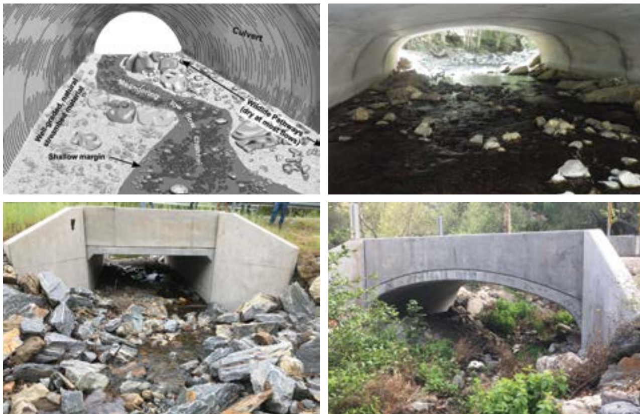
Figure 4.43—Stream simulation design and function moving through a culvert (top left, figure from Keller and Ketcheson [2015]) and various stream simulation installations. Upper right and lower left photos by Gordon Keller, lower right photo by Jonathan Berry.
