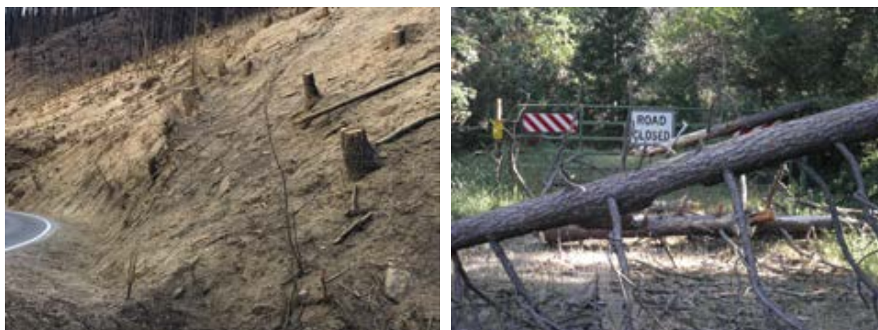
Figure 4.74—Hazard-tree removal site along a forest highway for traffic safety (left); other roads may remain closed because of hazard trees killed by drought, insects, and fires. Photos by Gordon Keller.
