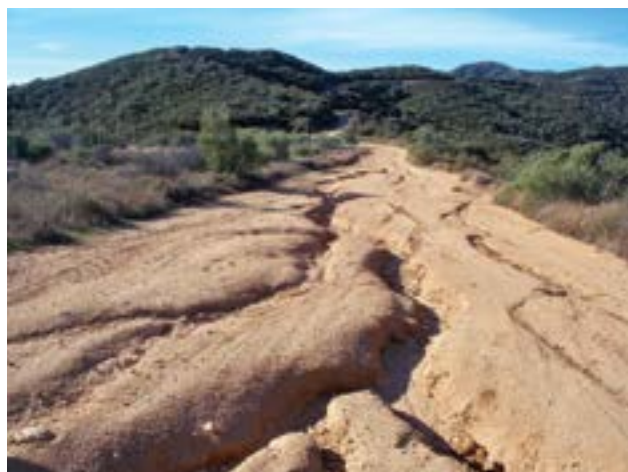
Figure 4.18—Ruts and erosion in the road surface due to lack of surface drainage and maintenance. These roads are particularly susceptible to damage from any storm when in this condition. Left photo courtesy of Joshua Direen; right photo courtesy of Vincent Barandino, USDA Forest Service, National Technology and Development Program.
