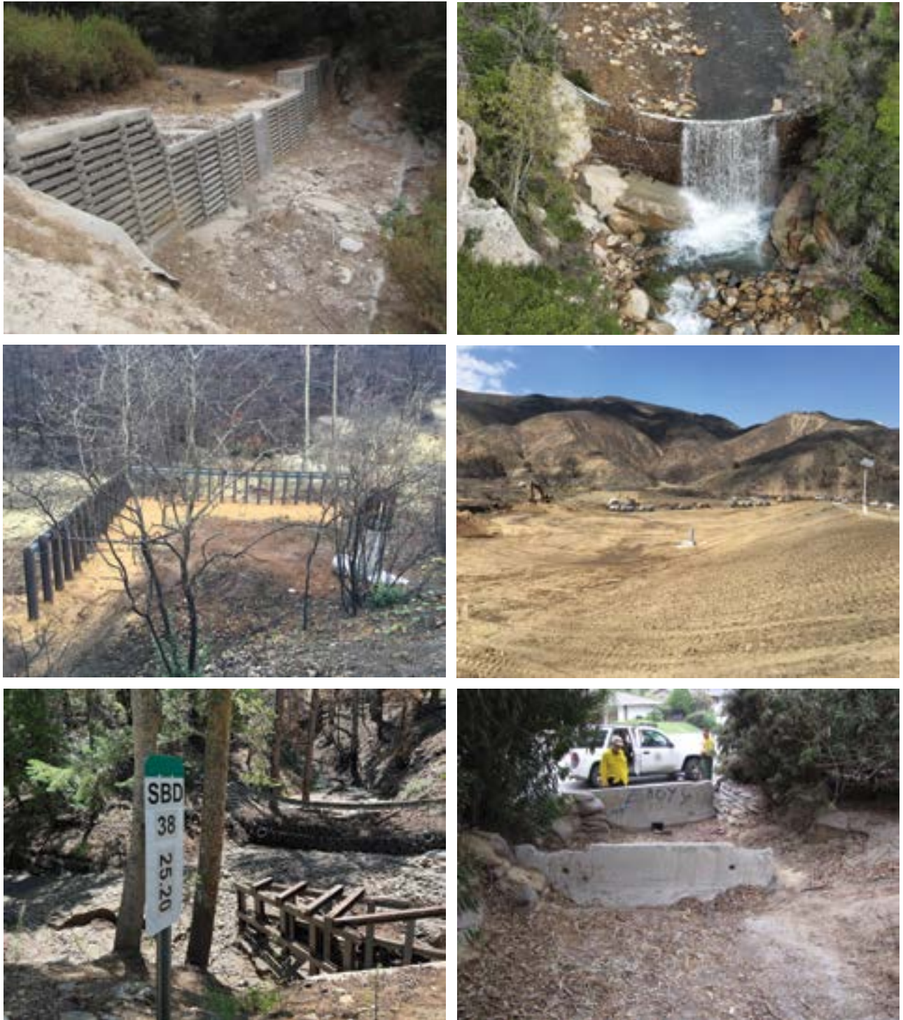
Figure 4.72—A variety of debris-flow retention structures or adaptation measures, including gabion walls, ring net structures, bollard and other debris racks, debris retention basins, channel modification and enlargement, and K-rail or structures to stop or deflect flows. Top left and bottom right photos by Allen King; top right photo by Yonni Schwartz; all other photos by Donald Lindsay.
