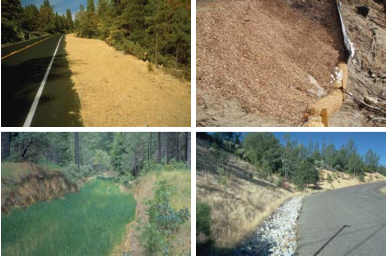
Figure 4.56—Common erosion control measures: (top) physical measures using straw mulch and netting (left), and application of woodchips and straw wattles (right) for ground cover and surface stabilization until vegetation grows. (Bottom) typical vegetative erosion control measures using grasses on a closed road (left) and deep-rooted shrubs and trees, as well as grass on a cutslope (right). Photos by Gordon Keller.
