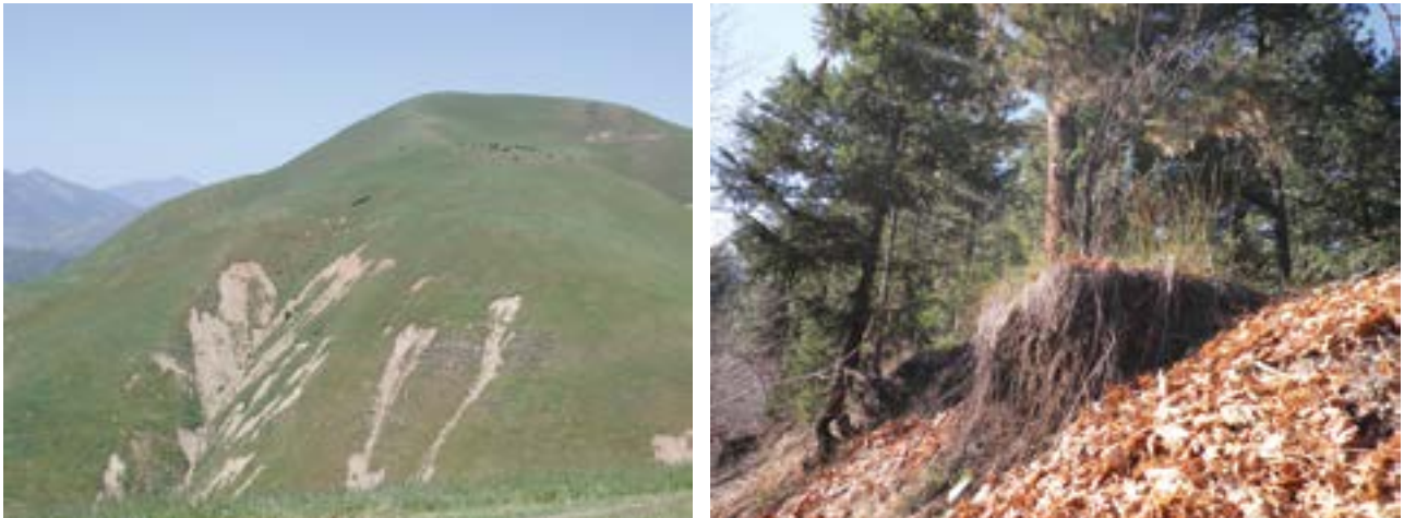
Figure 4.57—Slope failures from shallow rooted vegetation, such as some grasses. Photos by Gordon Keller.
