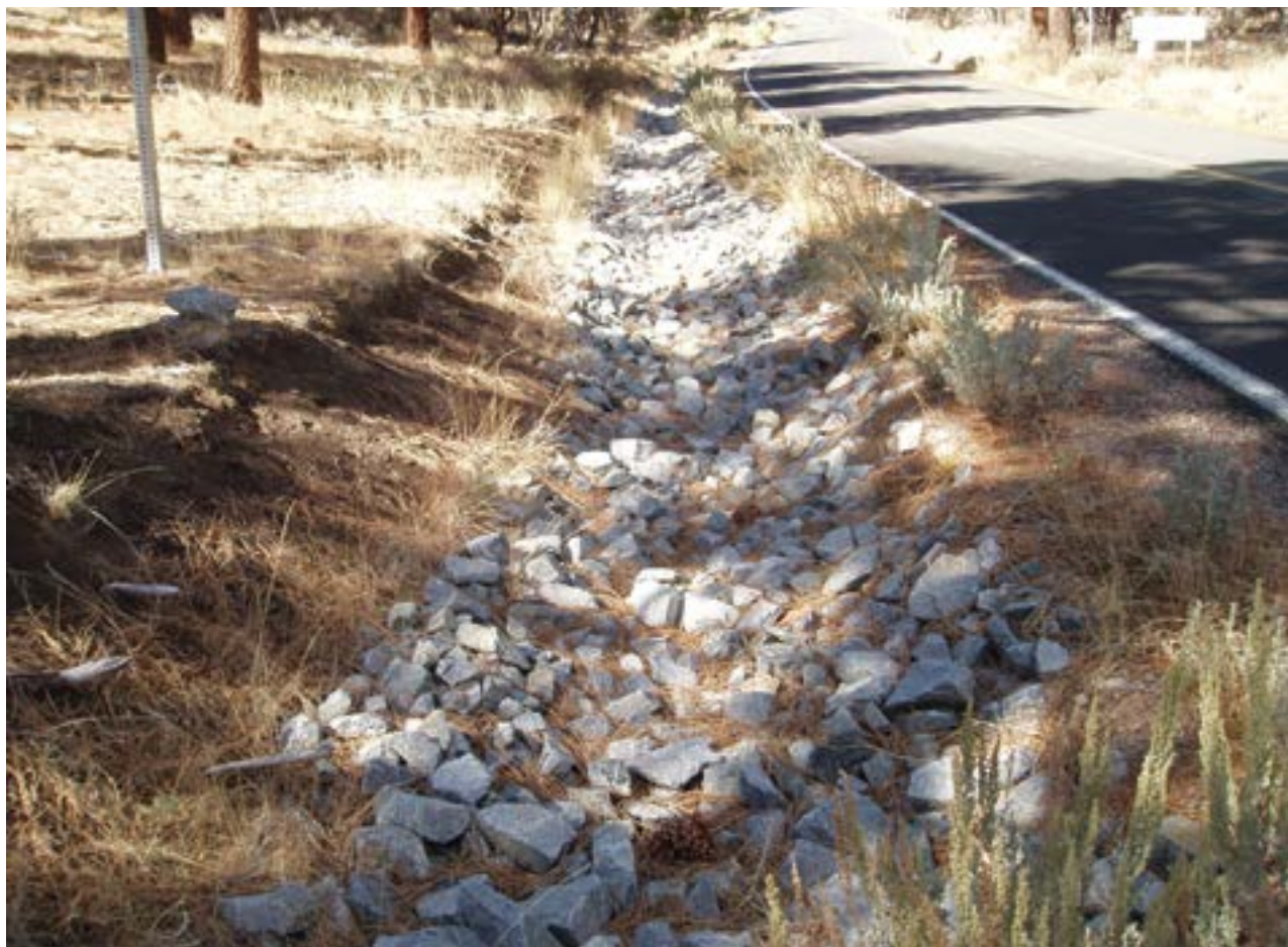
Figure 4.30—A rock-armored ditch to prevent downcutting and erosion of the ditch. Photo by Gordon Keller.
