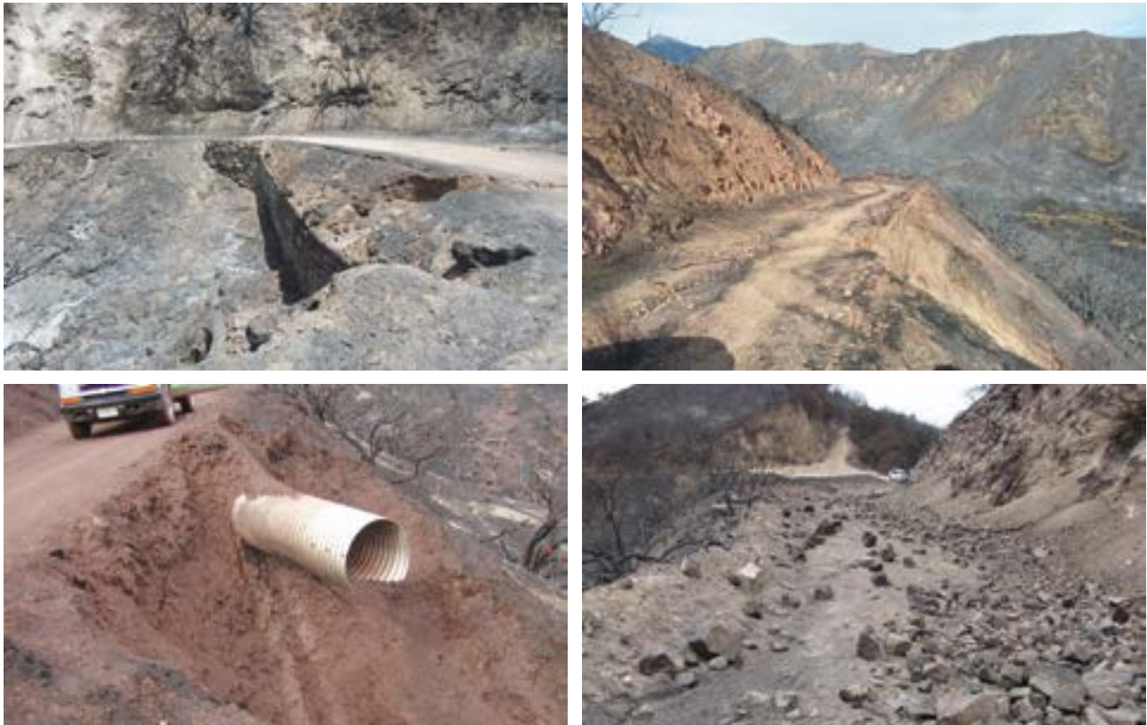
Figure 4.13—Postfire effects: as shown here, erosion rates increase, sedimentation problems persist, and fires followed by intense storms create frequent washouts, debris flows, stream debris torrents, rockfall, and landslides. Top photos by Joshua Direen, USDA Forest Service, San Bernardino National Forest; bottom photos by Allen King.
