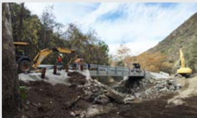
Newly constructed bridges and bottomless-arch culverts that have enhanced fisheries habitat and demonstrated to be resilient to flooding and debris flows. Photos show the Trabuco Creek crossing #3 after bridge construction (left) and Holy Jim #1 with a new bottomless arch (right).
