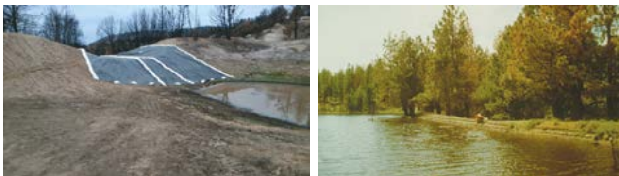
Figure 4.78—Earthen dams with minimal freeboard (distance between the waterline and the top of the dam) and risk of overtopping because of a blocked or inadequate spillway. In the left photo, the spillway is being lowered to create more freeboard. Left photo courtesy of Herman Wendell, right photo by Gordon Keller.
