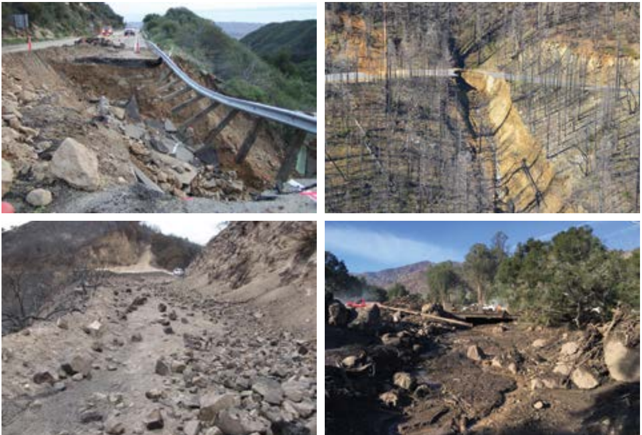
Figure 4.4—Landslides, slope failures, rockfalls, and debris flows that occur because of saturated soils from major storms and after wildfires. Left photos by Allen King, right photos courtesy of Donald Lindsay.
