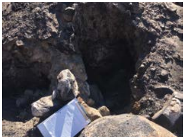
Figure 4.79—An earthen embankment of a dam where wildfire has burned the vegetation and tree roots, leaving deep voids in the embankment. This increases the risk of piping and dam failure, which can be mitigated by removing large vegetation from the dam face and embankments. Photos courtesy of Jonathan Berry.
