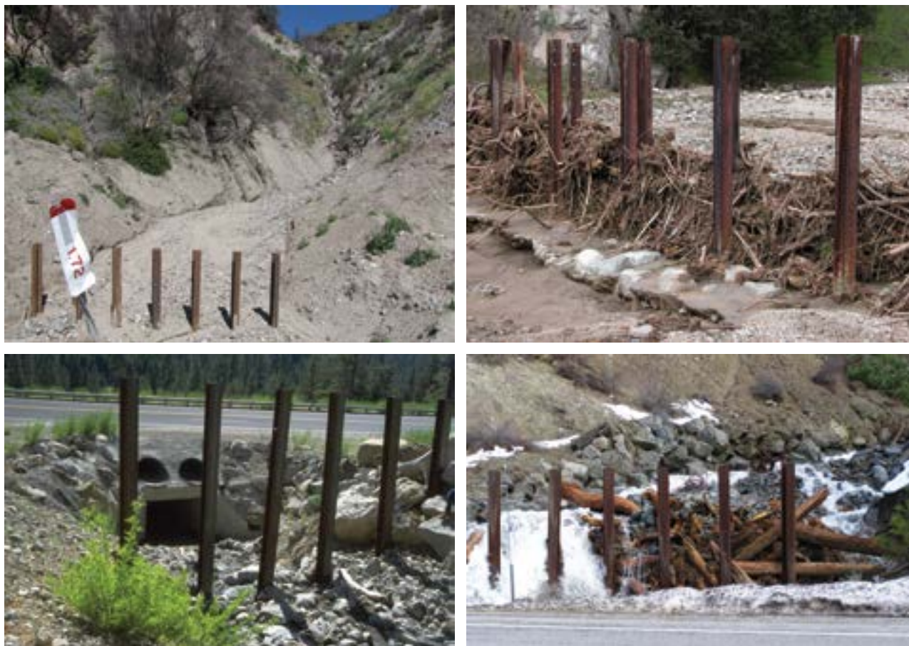
Figure 4.41—Bollard-type trash racks placed in channels or upstream of culverts before storms (left) and full of debris after major storms (right). Note that trash racks need to be cleaned periodically and maintained. Upper left photo by Allen King, upper right photo by Alan Yamada, lower photos by Gordon Keller.
