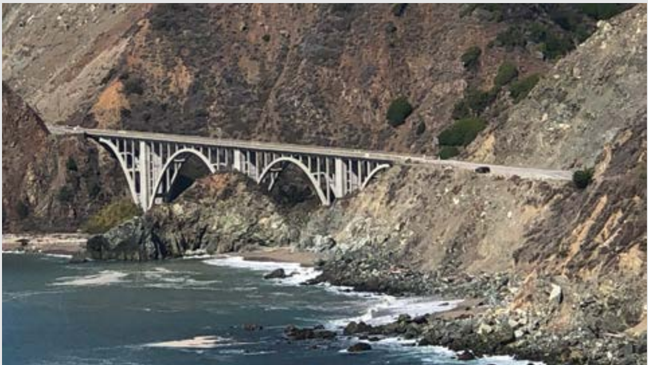
Figure 5.13—Big Creek Bridge, which was flagged by the California Department of Transportation as a high-priority bridge for climate change and in need of a detailed climate vulnerability assessment (Caltrans 2021). Photo by Lisa Wallace.
