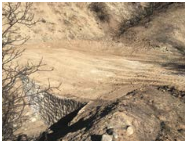
Figure 4.64—Slope stabilization structure types: a rock buttress (left) and an old masonry rock retaining wall (right). Left photo by Gordon Keller; right photo by Joshua Direen, USDA Forest Service, San Bernardino National Forest.
