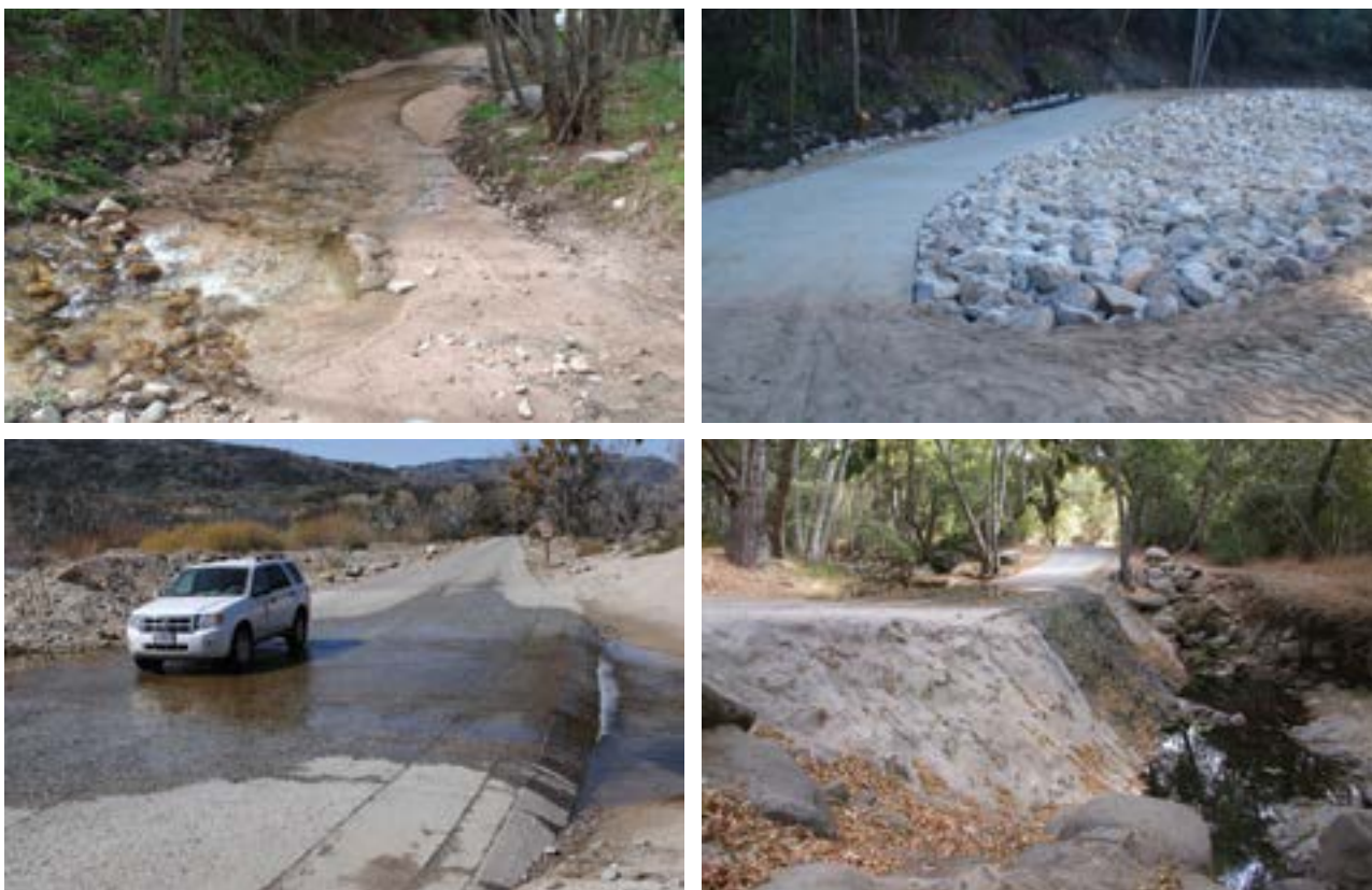
Figure 4.46—An old, unimproved ford (top left) and a new concrete slab ford (top right) on Deer Creek, San Bernardino National Forest. Bottom photos show two other armored fords. Top photos by Joshua Direen, USDA Forest Service, San Bernardino National Forest; bottom photos by Vincent Barandino, USDA Forest Service, National Technology and Development Program.
