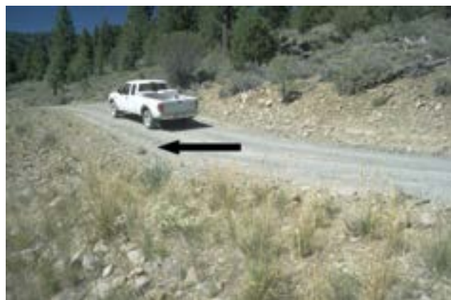
Figure 4.25—Installation of typical rolling dip cross drains on roads. Rolling dips are commonly used on forest roads to remove water off the road surface. They can also be used as a dip to prevent stream diversion down the road and direct flow back into the natural drainage. Left photo by Joshua Direen, USDA Forest Service, San Bernardino National Forest; right photo by Gordon Keller.
