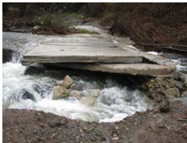
Figure 4.47—A ford damaged over time on Trabuco Creek, Cleveland National Forest, from downstream scour, or structure undermining. Upstream and downstream cutoff walls are typically needed to protect the structure. Photos courtesy of Kirsten Winter.
