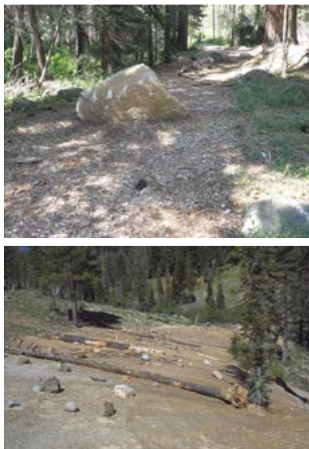
Figure 4.19—Road closure options include decommissioning (top), complete roadway obliteration (bottom), and storm proofing with measures such as outsloping, frequent waterbars or dips, and other treatments such that maintenance is not needed to prevent damage. Photos by Gordon Keller.
