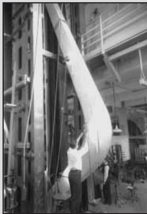
Glulam arches under test at the USDA Forest Service, Forest Products Laboratory in 1935.
