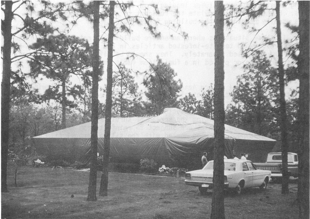
Figure 25. House covered with a gas-tight tarpaulin during fumigation for control of drywood termites.
