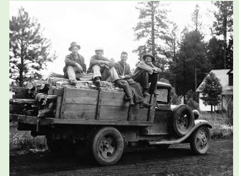
Sept. 1936—Juniper posts cut by Civilian Conservation Corps.
