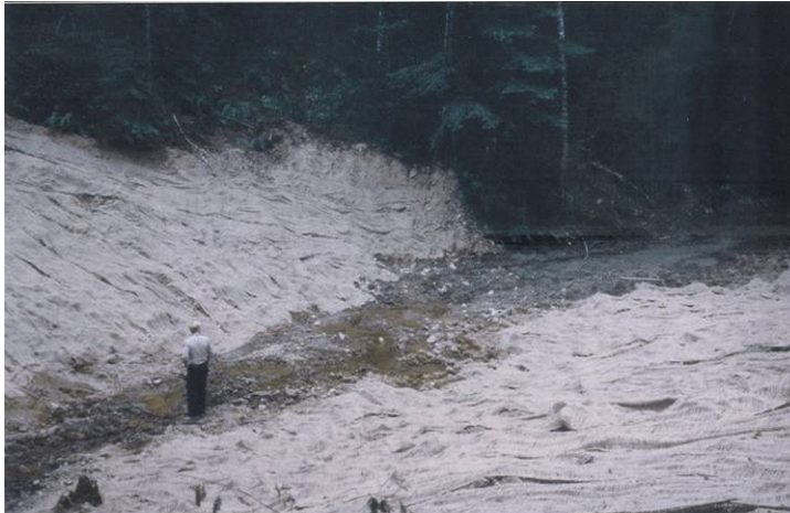
Figure 2. Excavated crossing CX-21 with jute netting on side slopes, November 1998.
