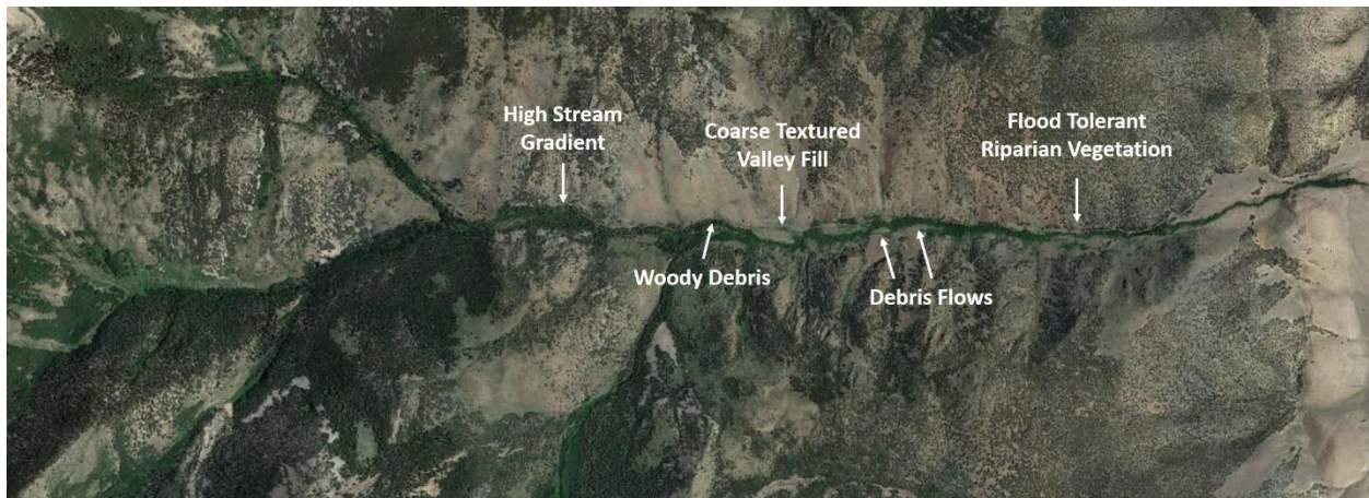
Fig. A.4.3 —Aerial photographs illustrating the geomorphic features in McCoy Creek, Nevada. McCoy Creek is a Type A 1 basin characterized by steep slopes and a relatively narrow valley floor. The channel is characterized by coarse sediment and woody debris and there is evidence of channel avulsion. Geomorphic characteristics are relatively consistent throughout this small watershed, and sample locations are selected at high, mid, and low elevations within the watershed. Image obtained from Google Earth on December 2, 2020.
