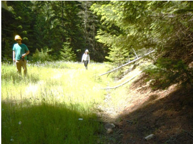
Figure 2c. Example of an overgrown road with no traffic in the Nez Perce NF (Elliot et al., 2018)
