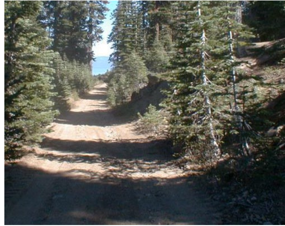
Figure 2b. Road condition that would likely be associated with harvesting, with wheel ruts and a large fraction of fines on the surface that will easily be detached by runoff (Villanueva, 2013).
