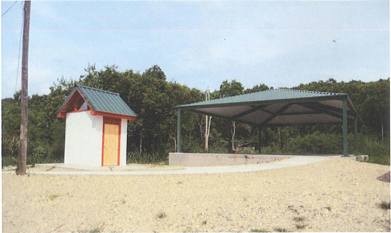
Figure 3. New facilities at Estate Thomas.
